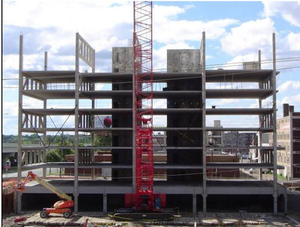
**Bookmen Stacks** condominiums in **Minneapolis, MN** utilized the recently patented ER-POST™ precast concrete truss system. The trusses span approximately 70' and are spaced at 40' o.c. allowing for large bays. Each truss has the ability to support two floors simultaneously allowing alternate levels to be completely column free.
