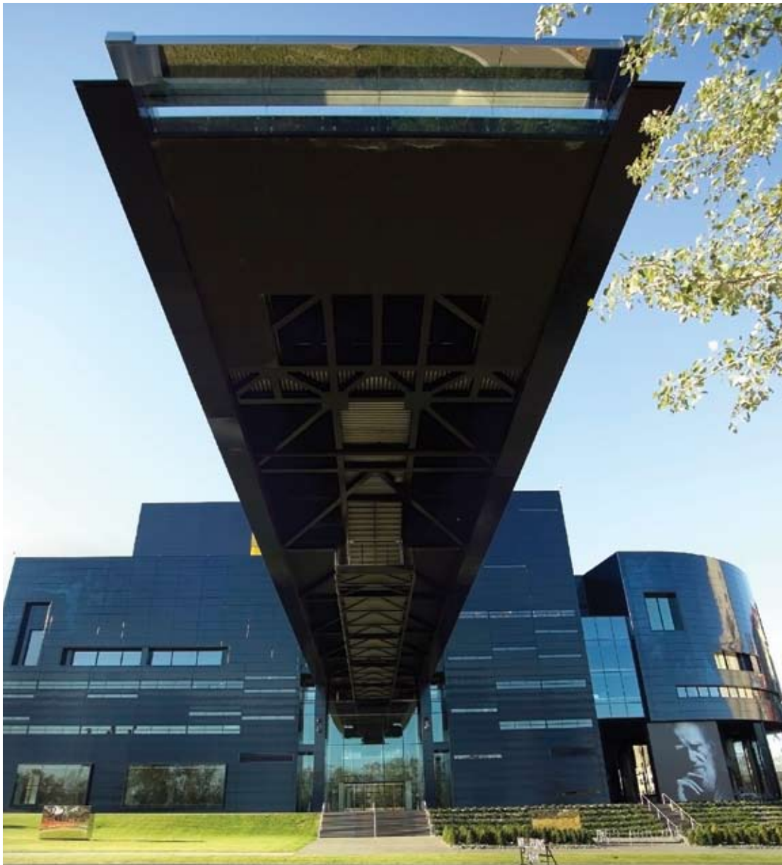
A catwalk beneath the endless bridge employs K-shaped braces similar to those used to support the cantilevered space itself. This bracing is exposed and, when lighted, lends aesthetic appeal to the form.
