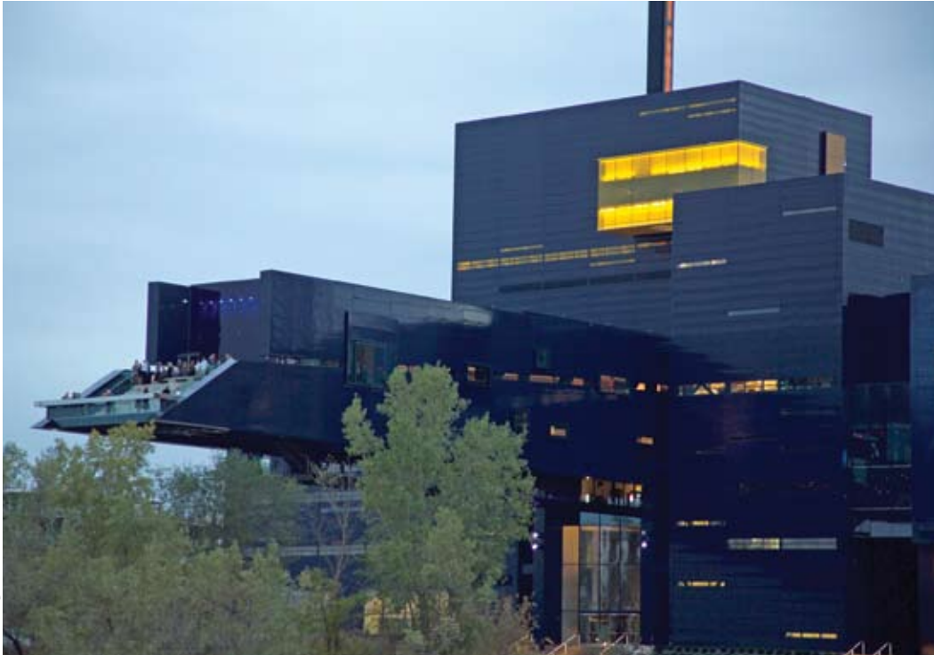
The endless bridge is covered near the building but is open to the sky at its end, with steps leading down to a safe viewing area. Inside, ramps lead from lobby areas to the cantilevered space.
